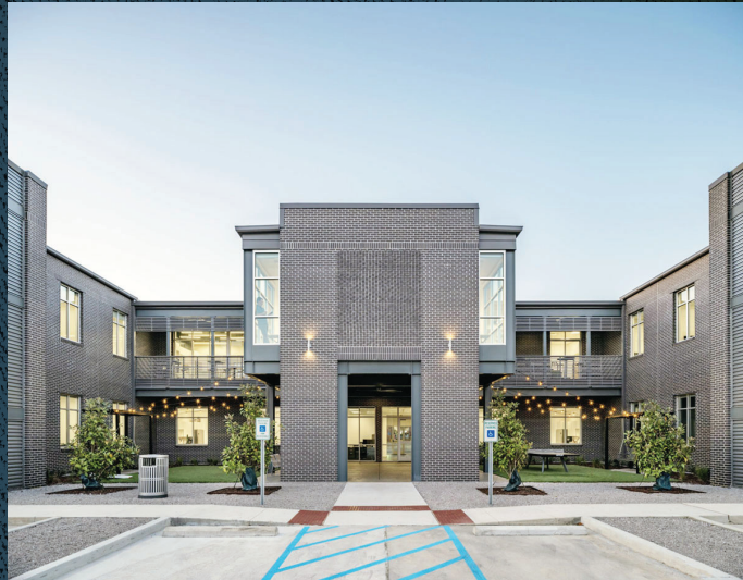
Stoa Group Headquarters Holly & Smith Architects
