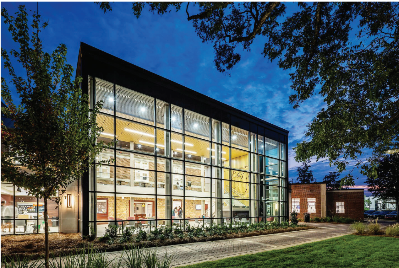
Renovated historic Perry Hall at Mississippi State University
